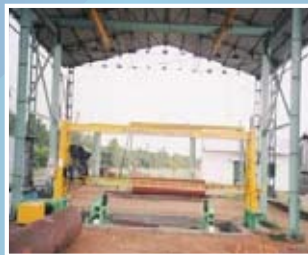
View of MS Plant
