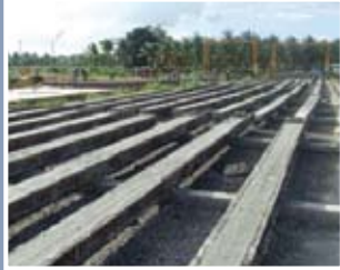
RCC Poles Casted
