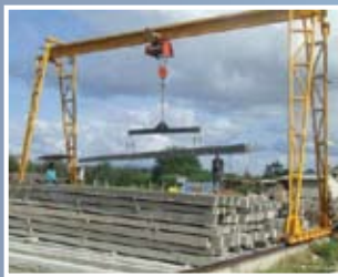
RCC Poles being stacked
