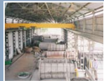
View of PSC pipes production lines
