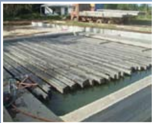
RCC Poles – Curing in Tank
